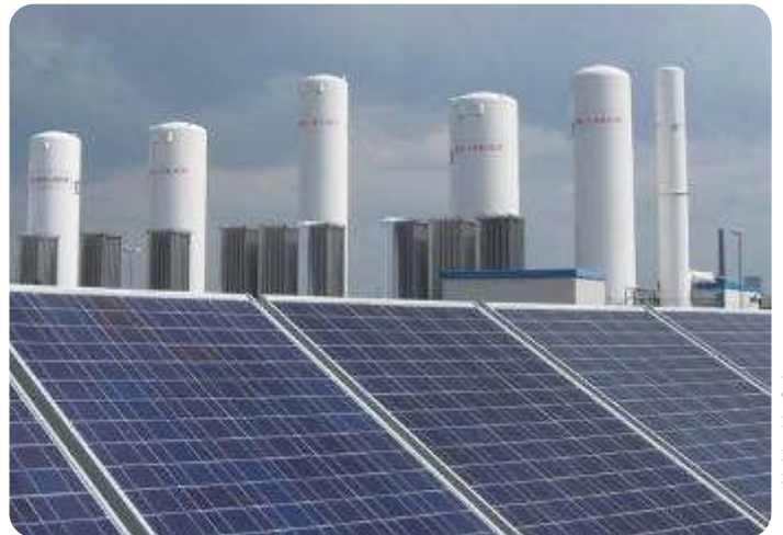
Air Liquide Solar
