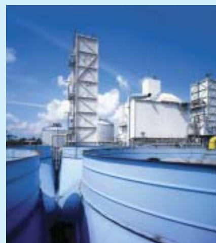
Air Separation Unit in Antwerp (Belgium)
