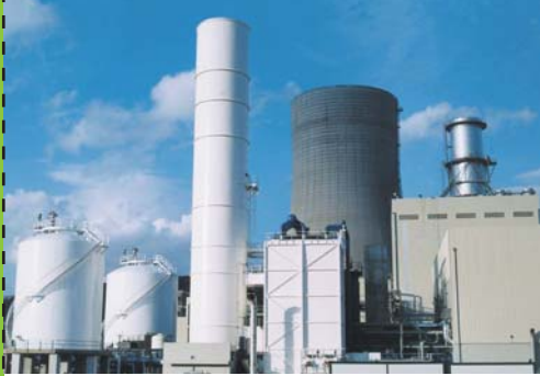
335 MW Elcogas project (Spain): full integration (heat, air compression, products). Today the only reference of this kind in the world.
