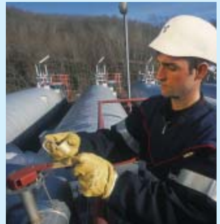
Carbon dioxide purification and liquefaction unit
