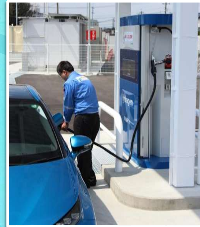
New hydrogen charging station
