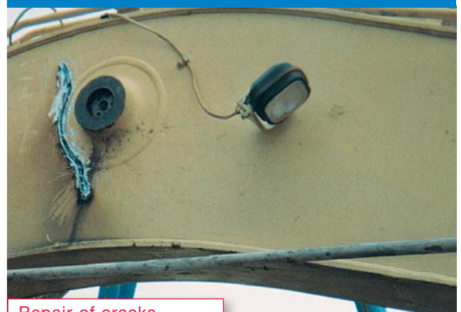
Repair of cracks
